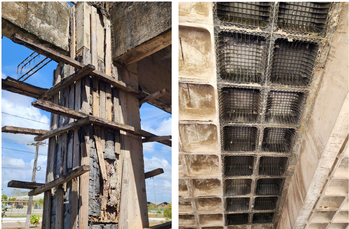
Figura 25: Pilar P24 e laje L8 com as formas
